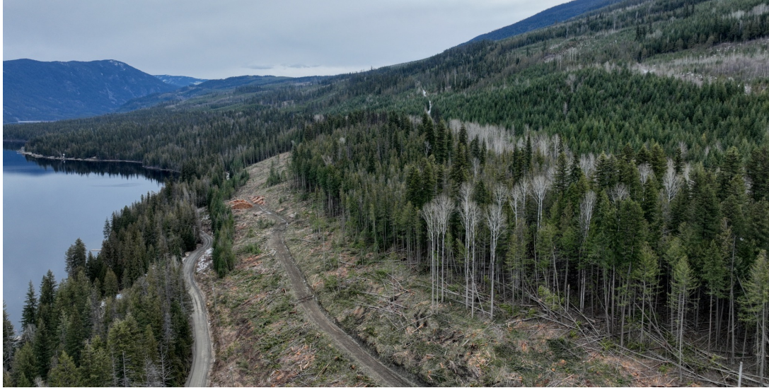
RW4 after winter harvesting. Piling, additional cleanup, and road rehabilitation are still planned.
